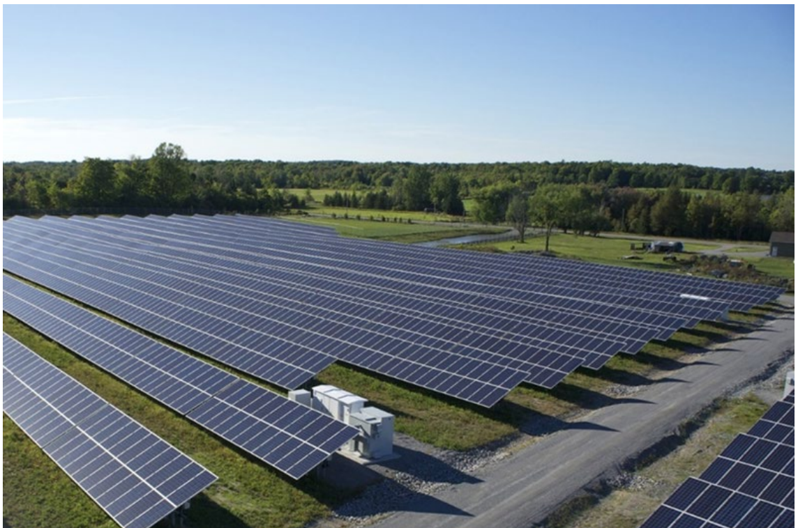
Image 4.2: Typical Fixed Panels (with Conversion Unit/Inverter)
