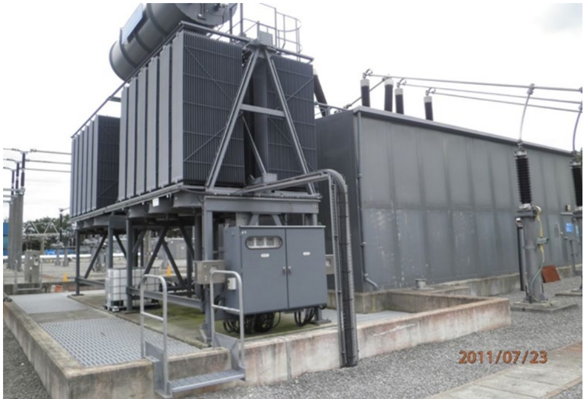
Image 4.5 Typical (large 400kV power transformer)
